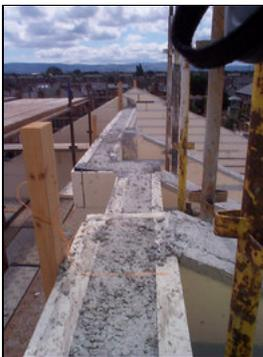
Polarwall was constructed off a concrete pad foundation. A mixture of open web joist floors and hollow-core planks were used together with a standard truss roof construction.
